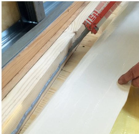
Bjælker påføres 3690 one-seal, for at fastgøre trinlydsdug.
